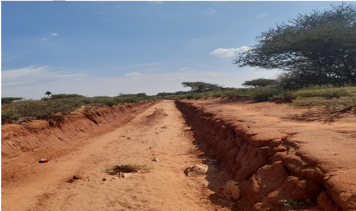
Figure 8. Critical deepening some section at existent route
